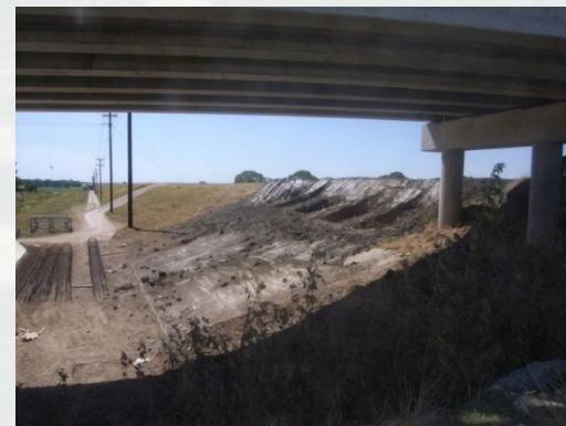
Levee raises and improvements
